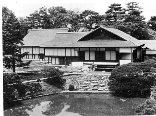
279 General view of shoin , Katsura Imperial Villa. 1620–4.
