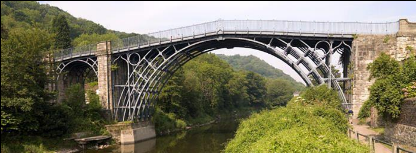
Abraham Darby III, Severn River Bridge, Coalbrook, England, 1779
