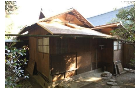
Sa'an Teahouse (Important Cultural Property), 1742 Gyokurin'in, Daitokuji, Kyoto
