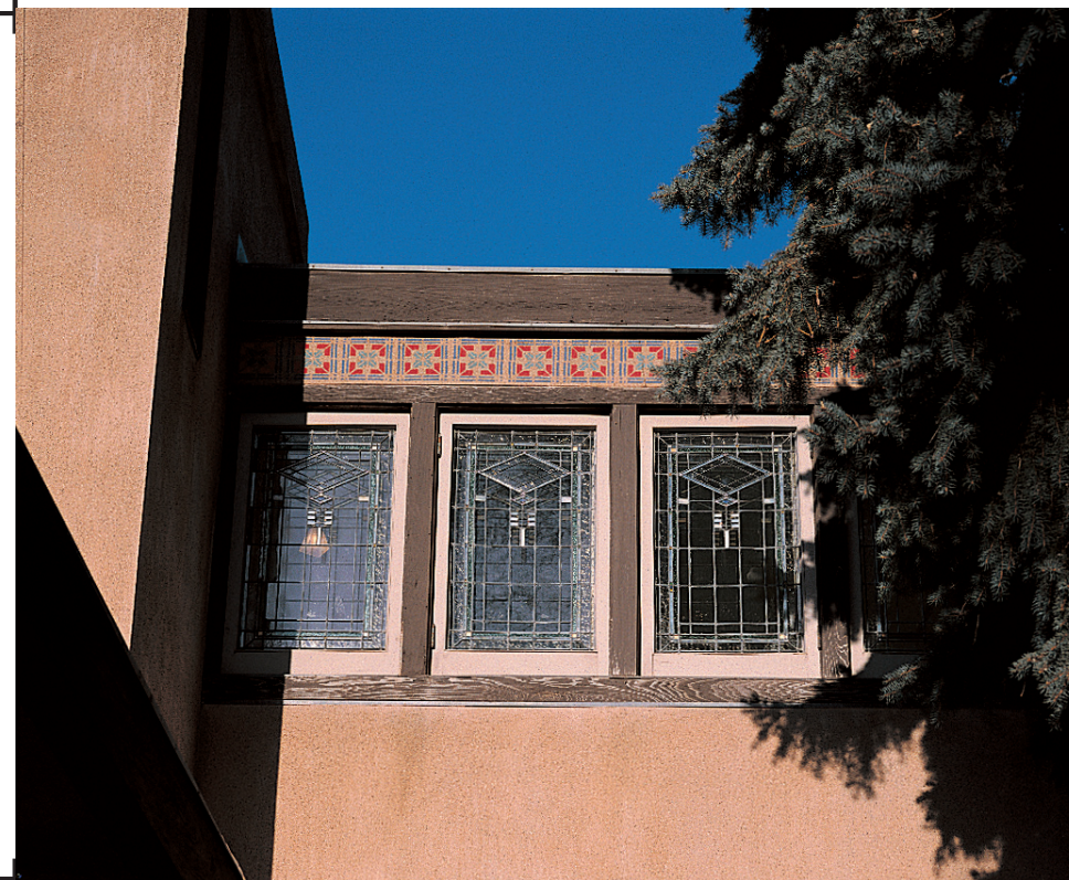
Second-floor windows and stencil Photo: Christian Korab
