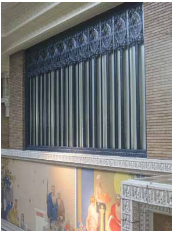
Mezzanine level of courthouse showing elevator-bank grille
