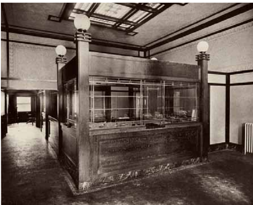
Teller booth with skylight, Madison State Bank Photo: William Gray Purcell Papers, Northwest Architectural Archives, University of Minnesota Libraries, Minneapolis
