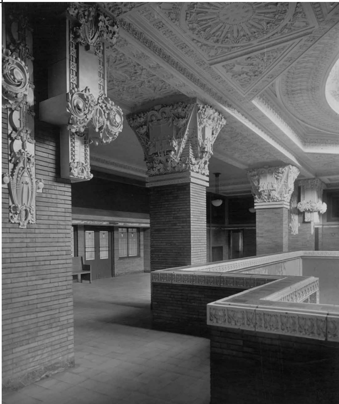
Woodbury County Courthouse, mezzanine with terra-cotta decoration, c. 1921
