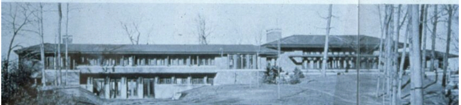
Wright, Francis Little House, Deephaven, MN, views from drive, c. 1914
