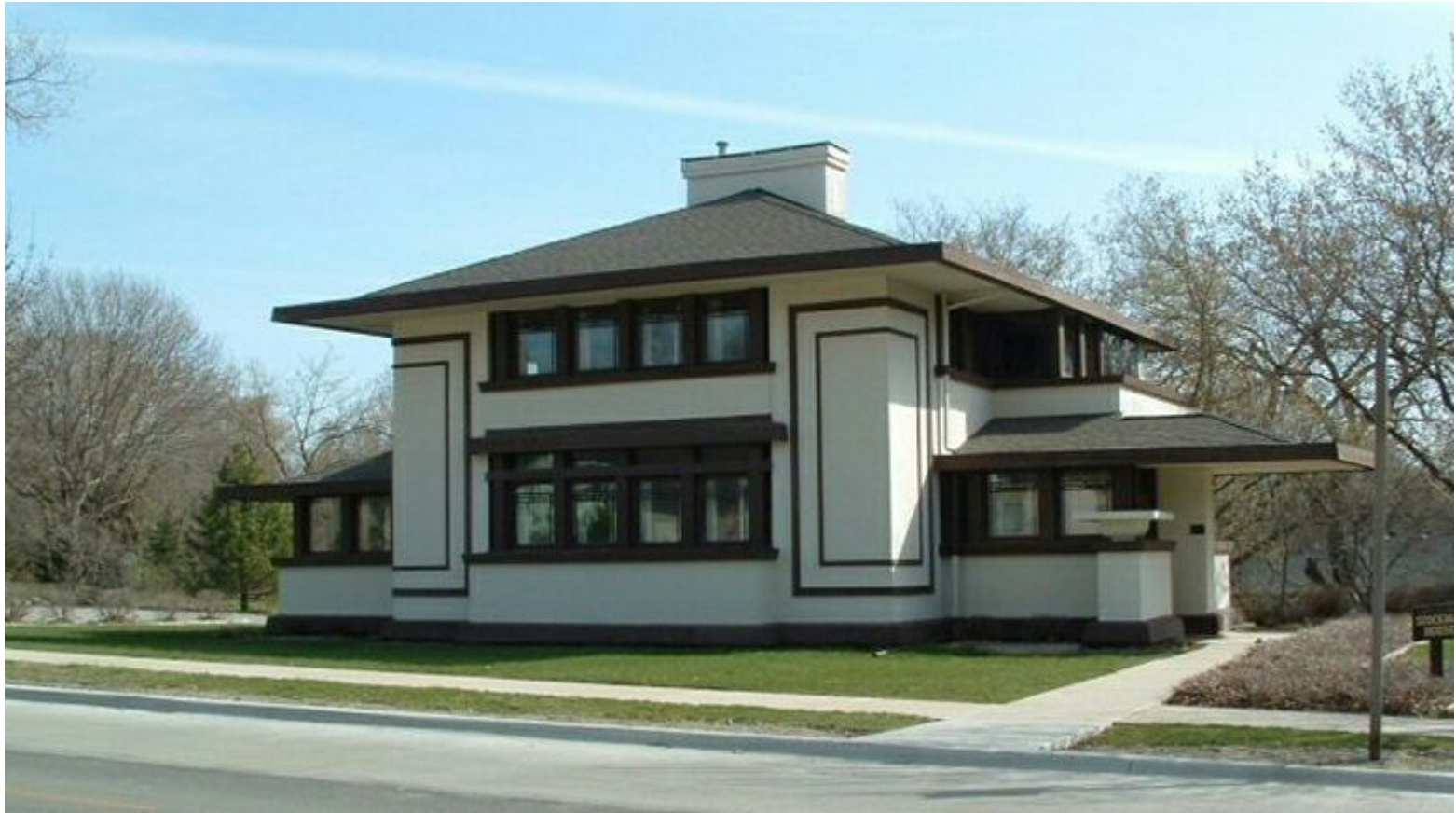
Wright's "Fireproof House" and Stockman house, Mason City, IA, 1908
