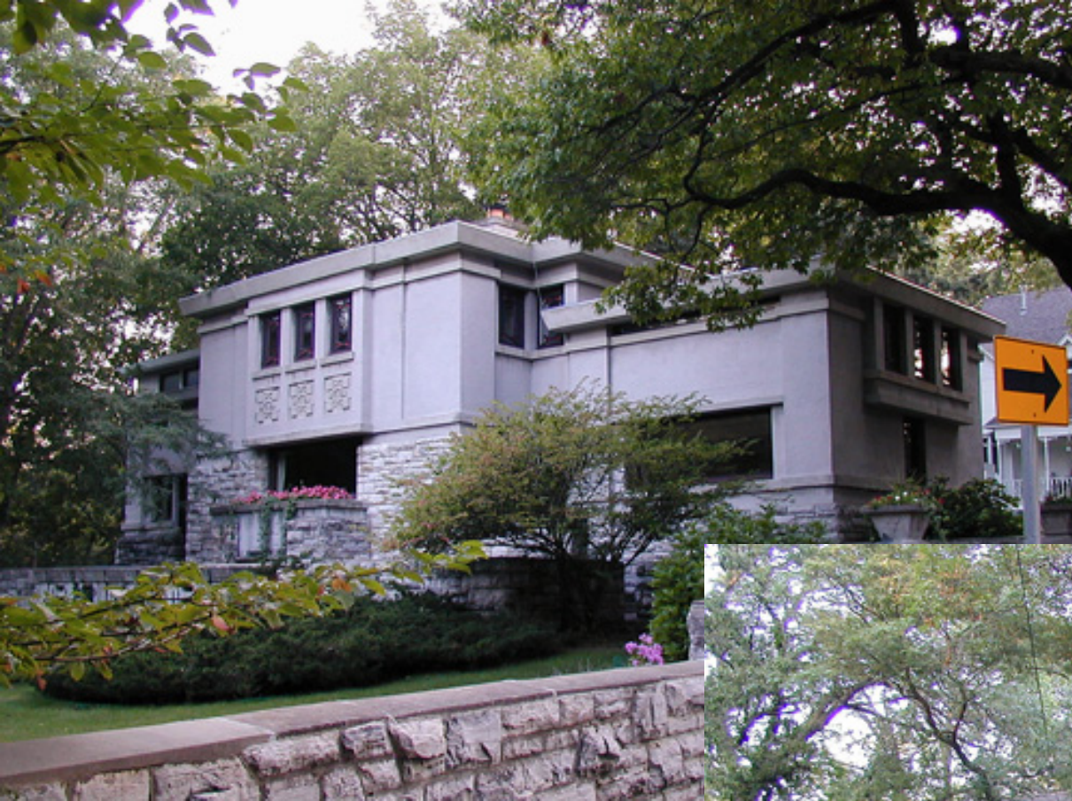
Walter Burley Griffin, James C. Blythe House, 1913, and Harry D. Page House, 1912, Walter Burley Griffin, Mason City, Iowa
