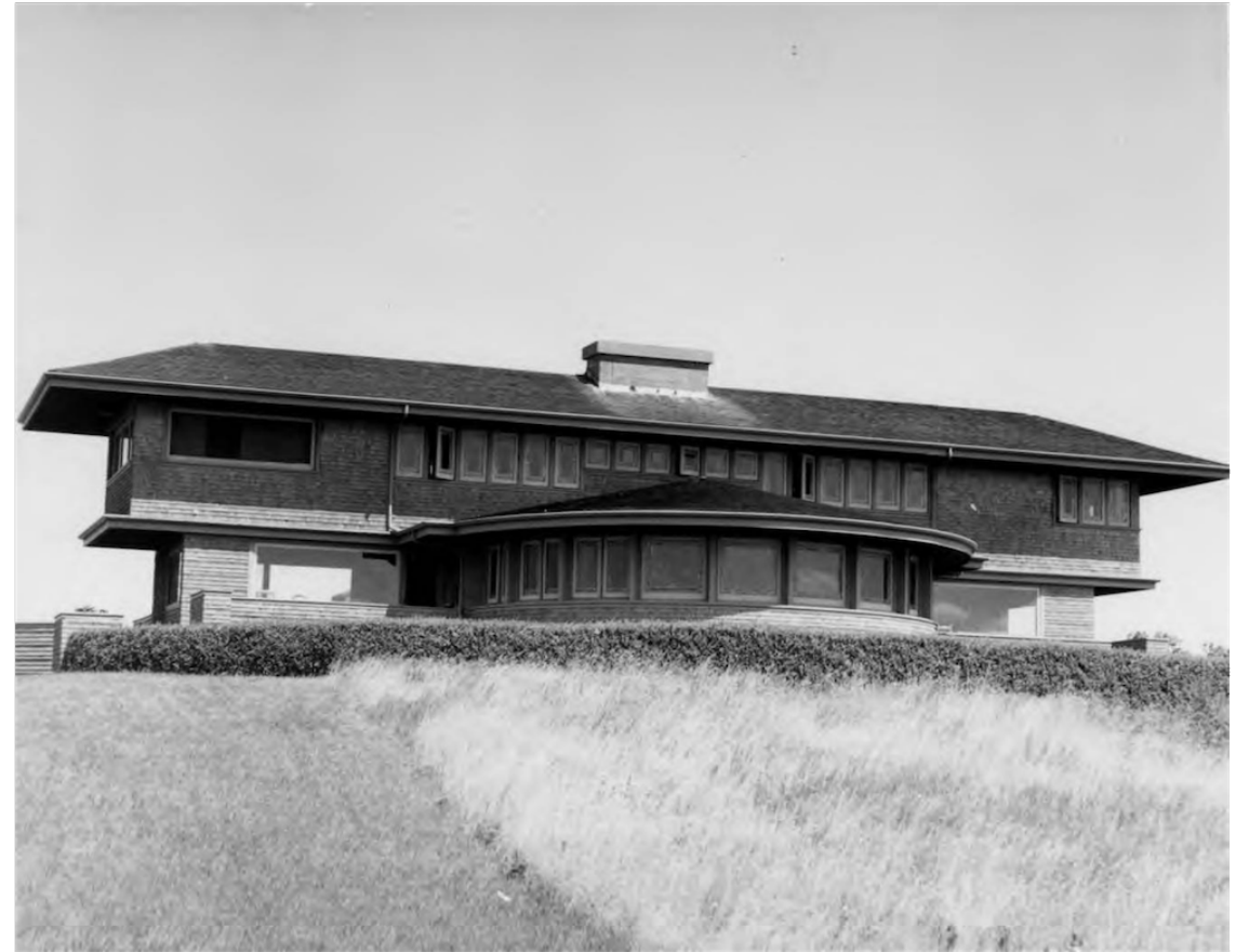
Bradley Bungalow, Woods Hole, MA, 1911, sleeping porch 2 nd floor left
